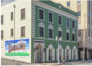
RAMP offices are located in the Gill Memorial Building in downtown Roanoke, VA
